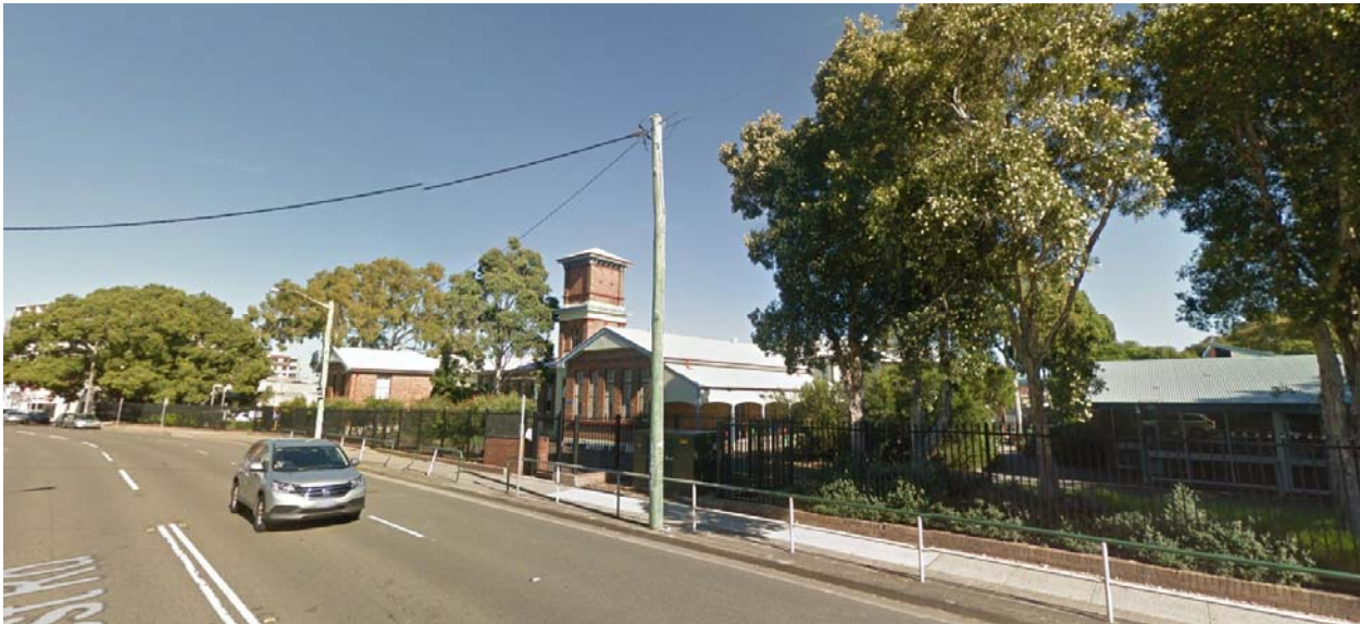
Figure 15: View along Forest Road of Hurstville Public School (Source: Google Maps)
