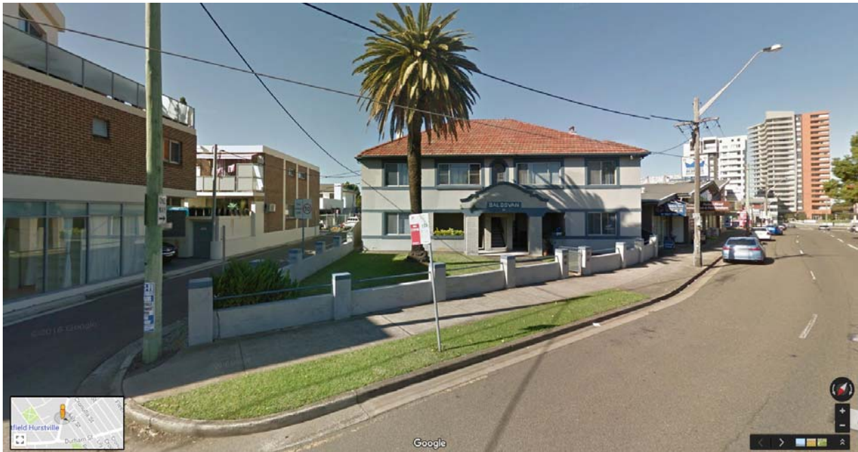
Figure 8: Site photo showing residential flat building on the corner of Forest Road and Roberts Lane (Source: Google Maps)
