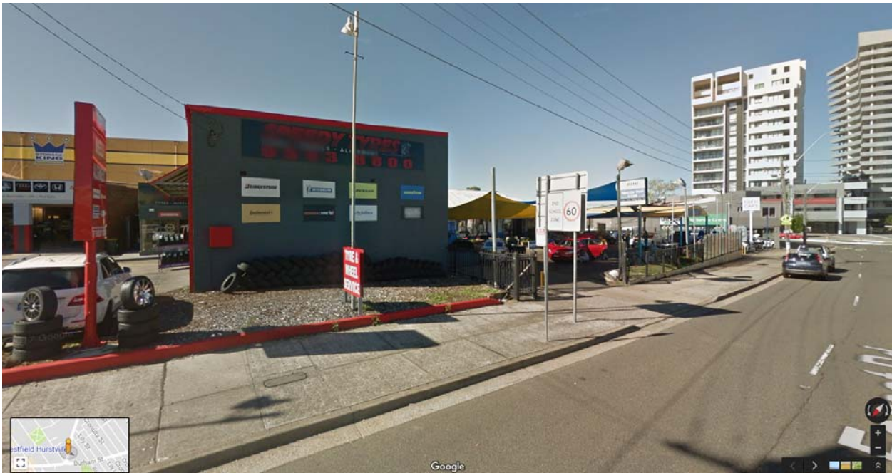
Figure 10: Site photo showing retail and commercial premises along the Forest Road frontage looking south (Source: Google Maps)
